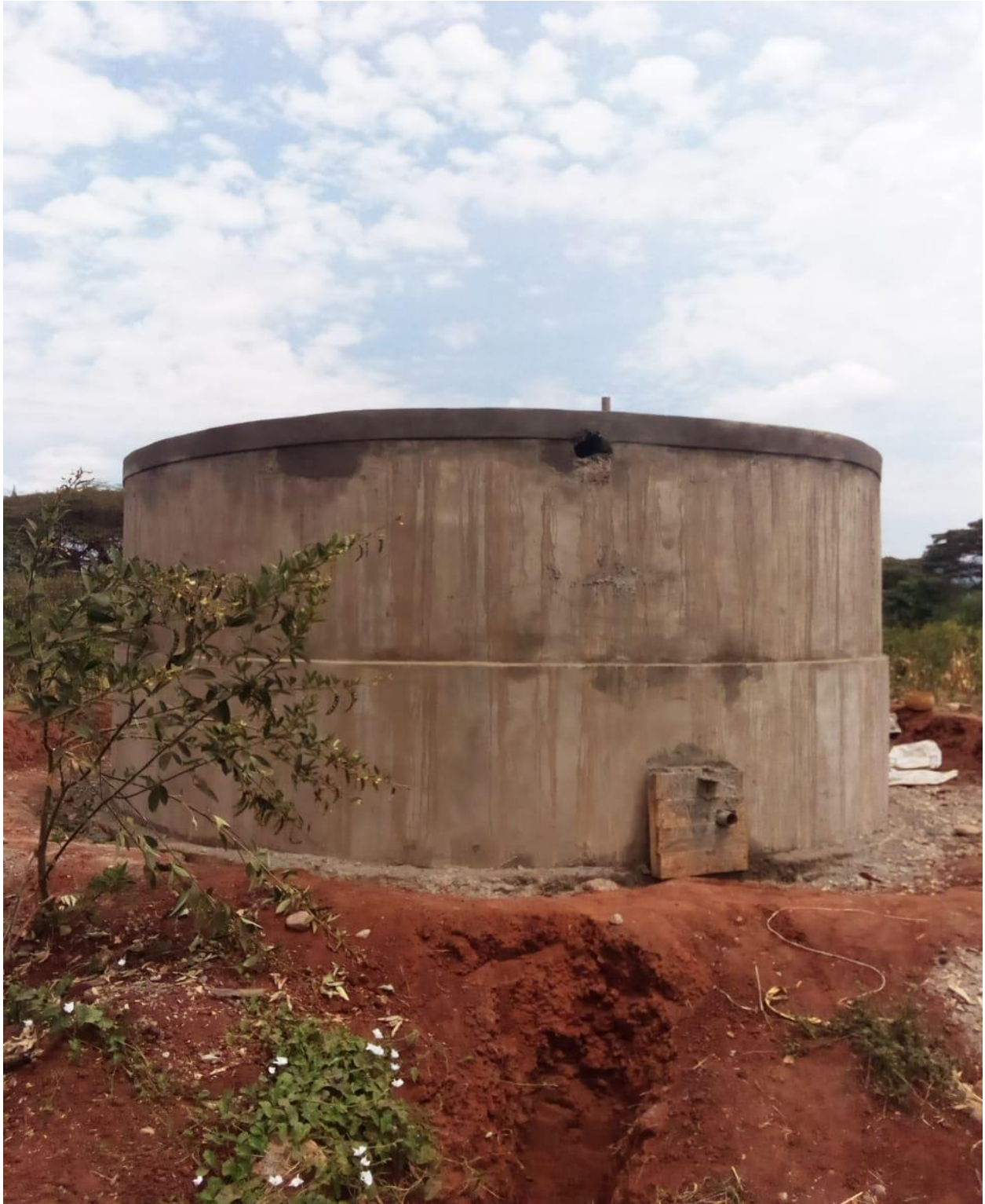
Masonry tank during construction
