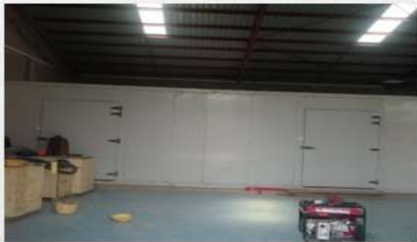
Refrigeration chambers at Kalongo cold store
