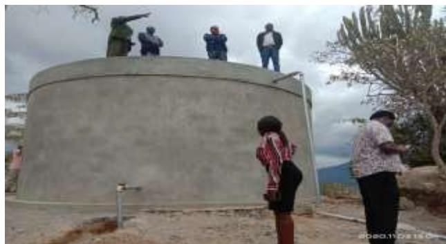
Masonry storage tank
