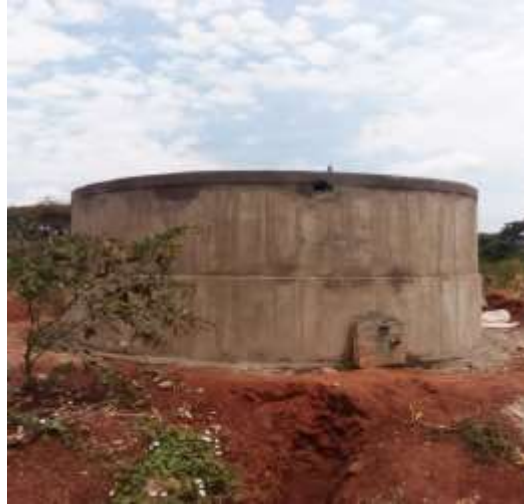
Masonry tank during construction
