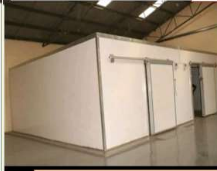
10 Tones capacity refrigeration chambers at kavuthu
