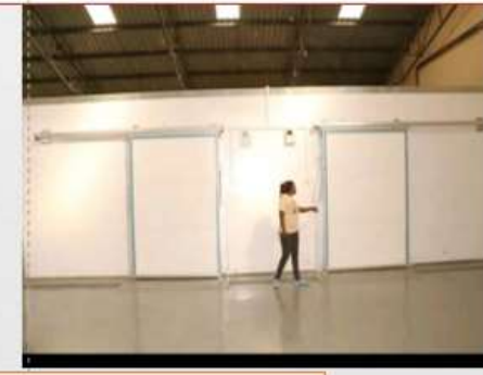
10 Tones capacity refrigeration chambers at kavuthu
