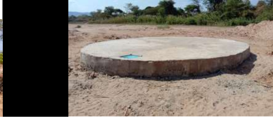
Project intake sump tank at the river
