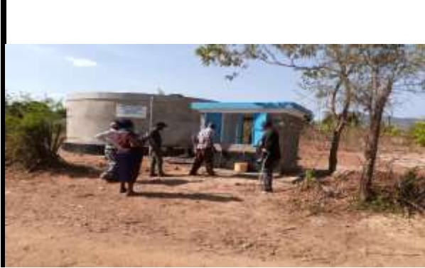
Project masonry tank 100M3 and water kiosk no. 1 in operation
